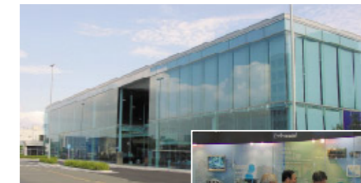
New pavilion "AISIN com-center"
