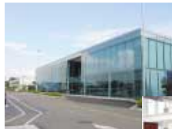
New pavilion "AISIN com-center"
