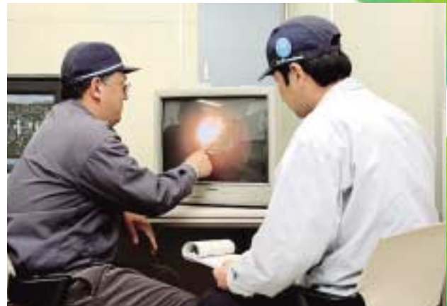
Checking the combustion status in the furnace at the centralized monitoring room in the waste incineration facility
