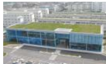
Rooftop of Aisin Com-center
