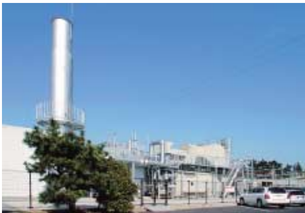
Entire view of the Nishio cogeneration system
