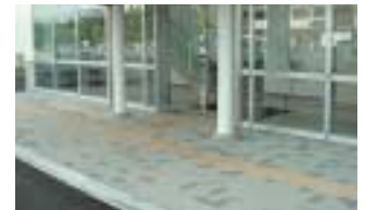
Permeable brick promenade in the new Kariya Plant
