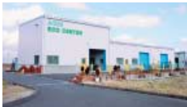
External view of the Aisin Eco-center
